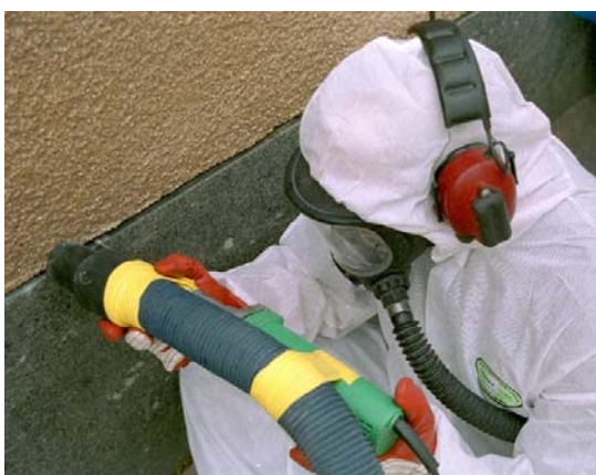
Grinding with a grinding pin and dust collection close to the tool.
