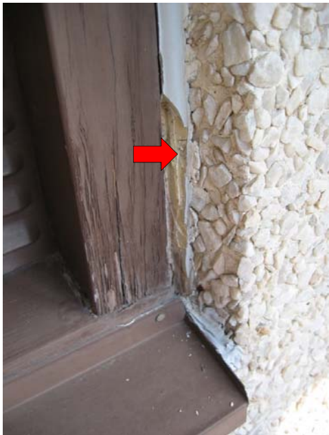
Sealant adjacent to window
