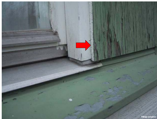
The sealant is concealed behind the panel
