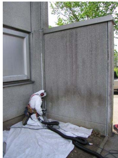
Oscillating knife cutter from Fein, model FSN 400E with the SP dust collector and Riktaflex.
