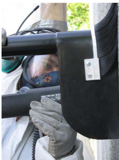
Grinding joint walls with the Milwaukee AGV 16180 QXC grinder, equipped with the SP dust collector.
